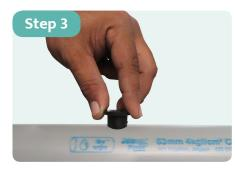
Insert the Top Hat Grommet fully. Ensure that the collar is resting on the pipe wall.
