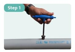
Use drill size of 17.5 mm to make the drill hole on the pipe.
